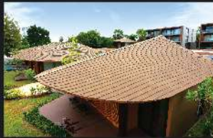
Veyla Cha Am, Phetchaburi Designed by: Architects 49
